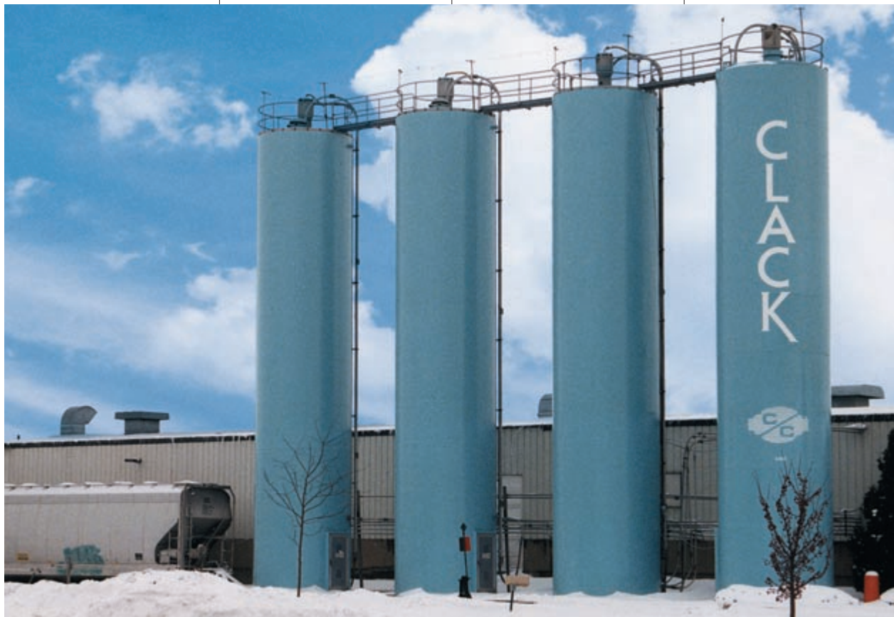
Here's a typical pellet transfer with a plastic pellet car ready for unloading. Walthers Archives
