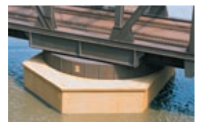
The center pier is tapered so water flows around it easier. This helps keep water currents in the boat channels in check and helps prevent debris from sticking on the pier.
