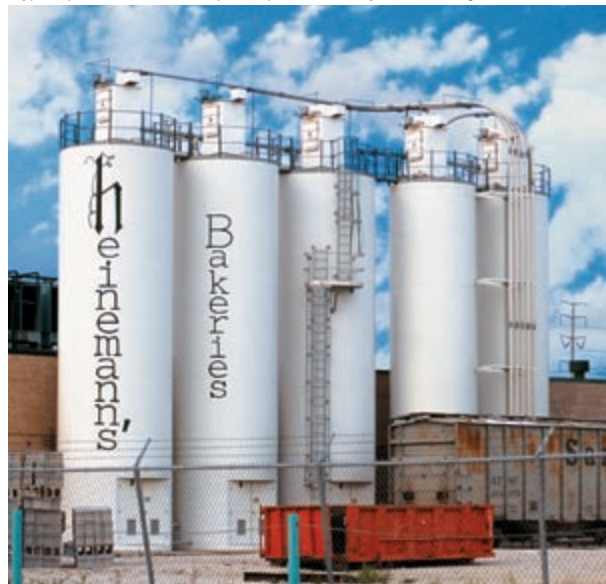
Heinemann's Bakeries in Chicago uses a similar facility for unloading bulk flour from Airslide® hoppers. Photo by Bob Gallegos
