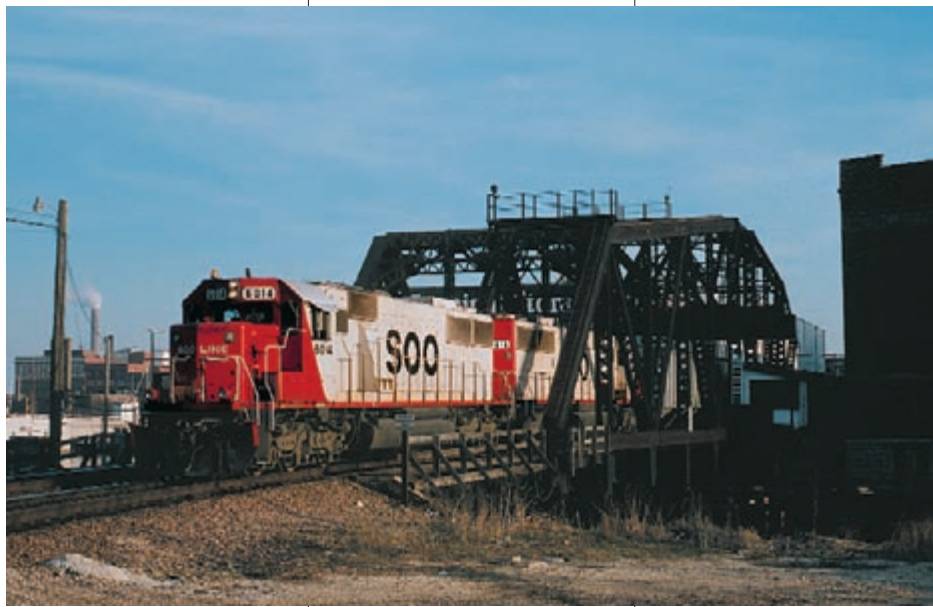
The Canadian Pacific's former Milwaukee Road swing bridge in Milwaukee. The pivot is off-center and the span is counter weighted. Photo by Bob Gallegos
