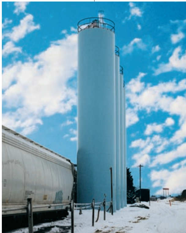
Here's a view of the piping system along the tracks. Walthers Archives
